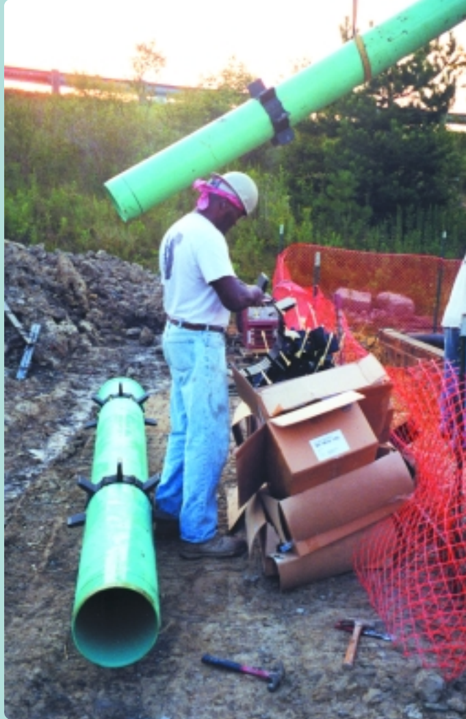
A worker installing MIDI Ranger II casing spacers on pipe sections.
