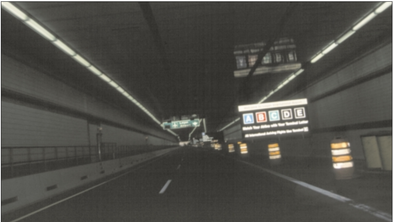
Rebuilding multi-level interchanges and constructing new tunnels and bridges entails some of the most detailed ITS-related applications.
