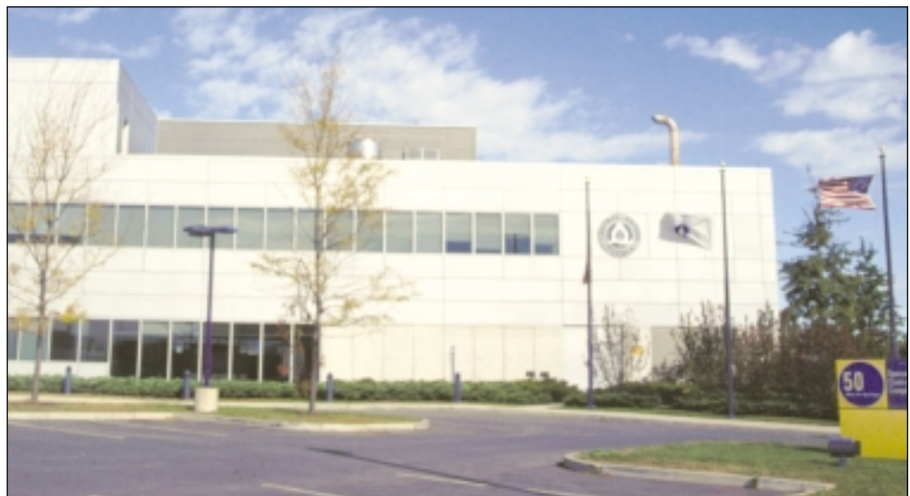
The Operations Control Center receives and processes data from a full spectrum of ITS applications.
