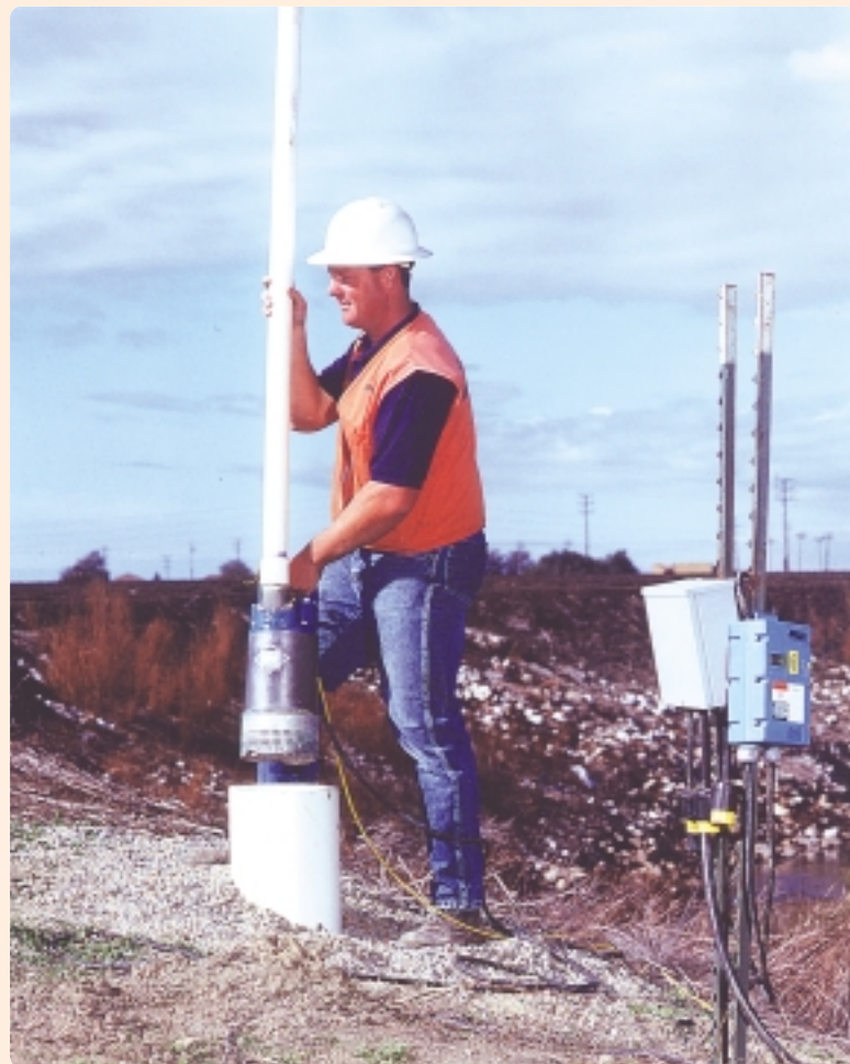
The pumps were easily pulled from the wells when an area was drained and advanced to wells drilled in the next work area.
