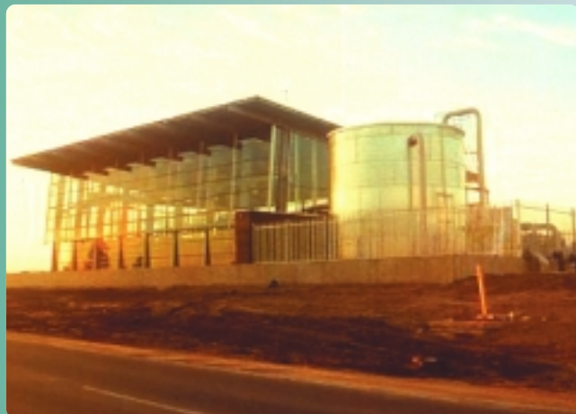
Left: The wastewater reclamation plant that recycled sewage and rainwater runoff at the Sydney Olympic Games Site in Homebush Bay, west of Sydney. The purification process involved the use of reverse osmosis (RO) technology.
