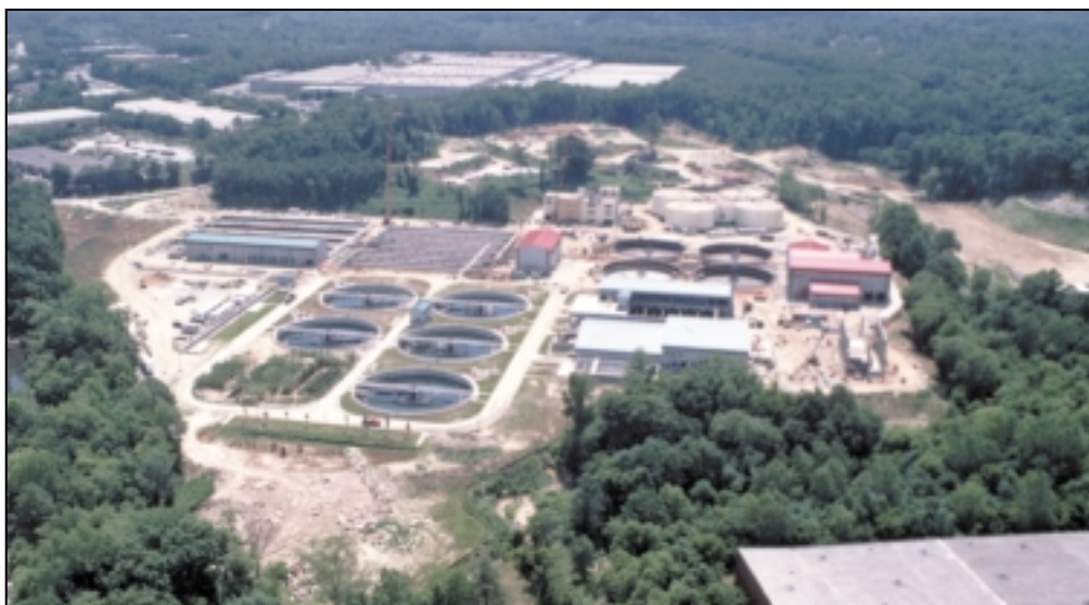
Utoy Creek Water Pollution Control Facility (WPCF).
