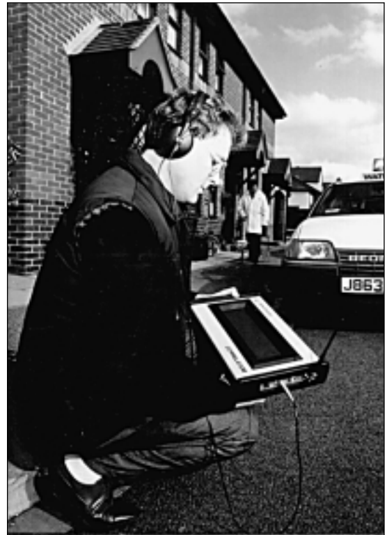
Using a leak noise correlator, an engineer can quickly locate a suspected water leak in a city street.
