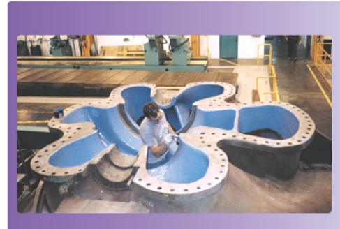
Used to repair a worn and leaking coolingwater pump, Devcon products helped it to be returned to service in less than two weeks. After sand blasting, washing, and priming the huge pump's inner walls, workers filled cracks, pits, and holes with Devcon Titanium Putty. For long-term protection, internal surfaces were then coated with Devcon Brushable Ceramic (shown here) to produce a smooth surface that resists corrosion and abrasion.
