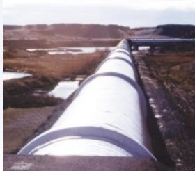
▼ Portions of the 8,800′ pipeline were elevated 20′–25′, making this project particularly challenging.
