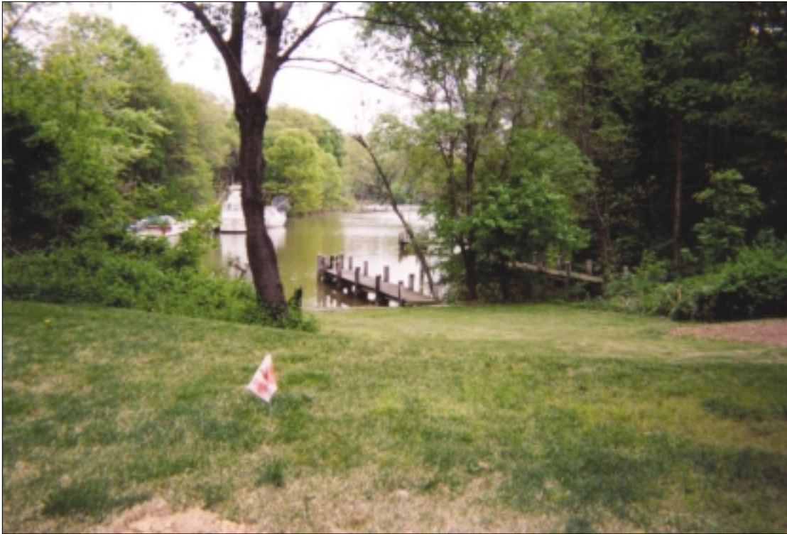
Figure 1: Sewer Outfall Flowing From Right to Left Under the Centerline Indicated by the Flag
