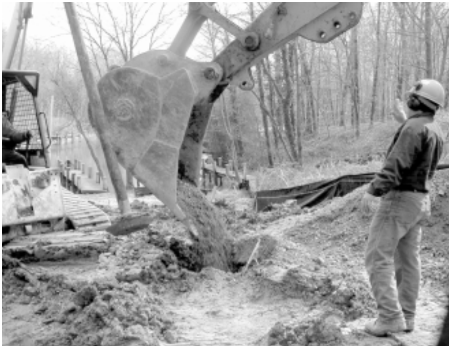
Figure 3: Geopier Installation
