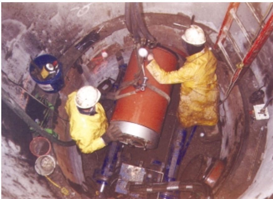
Sewer construction using pilot tube technology provides a safer alternative to open trenching.
