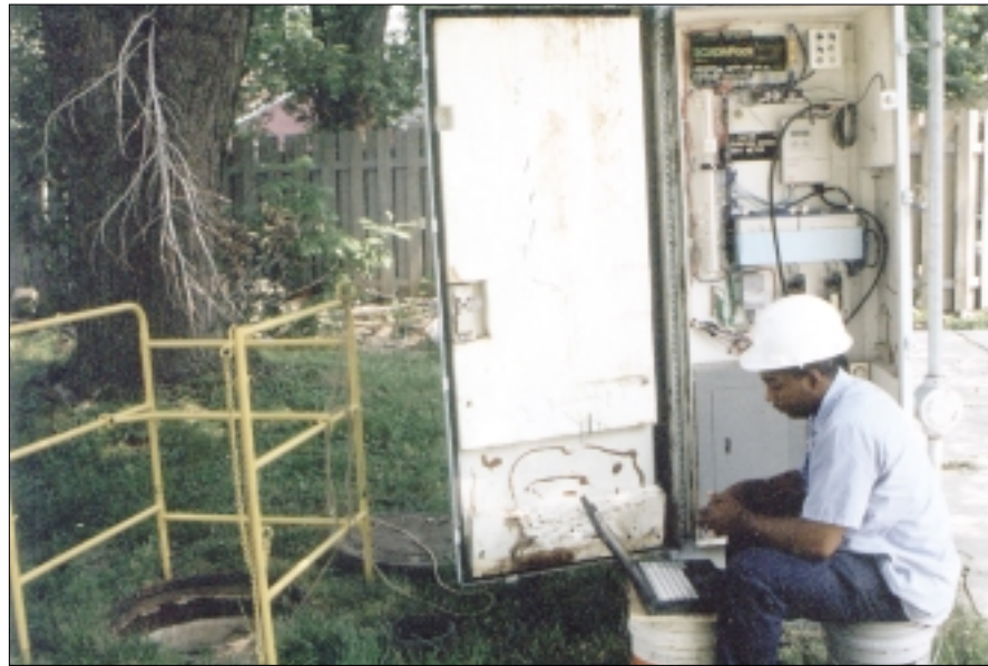
Figure 2: A technician sets up a portable PC for a CalMaster test run at a remote metering station.
