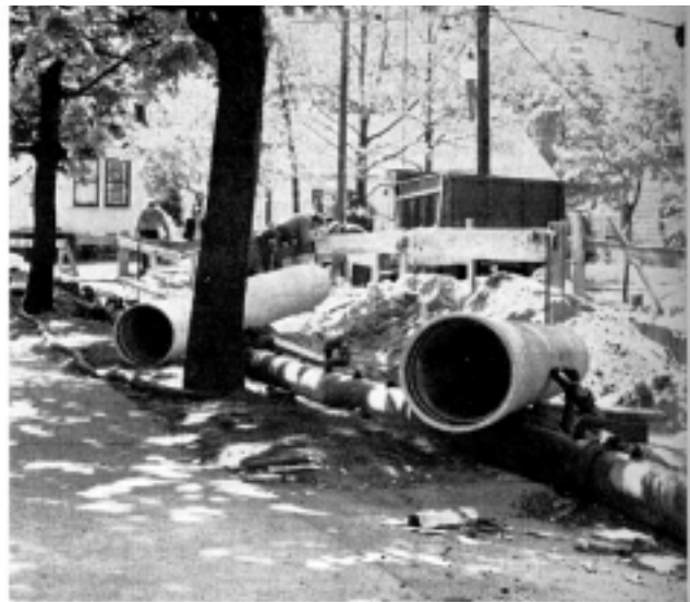
Well-point dewatering system along fully-sheeted trench for 24-in. asbestos-cement sewer pipe.
