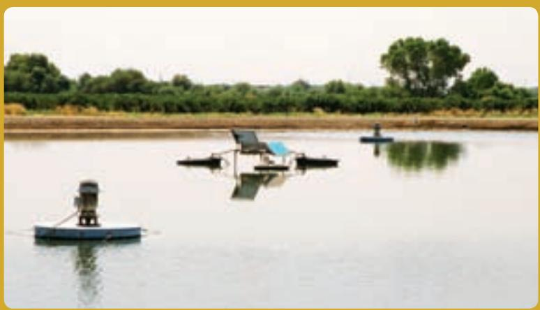
thorough pond mixing provided by SolarBee, with its long-distance high flow, provides effective aeration and significant reduction of biochemical oxygen demand (BOD), total suspended solids (TSS) and ammonia. It also solves odor problems and reduces sludge buildup.
