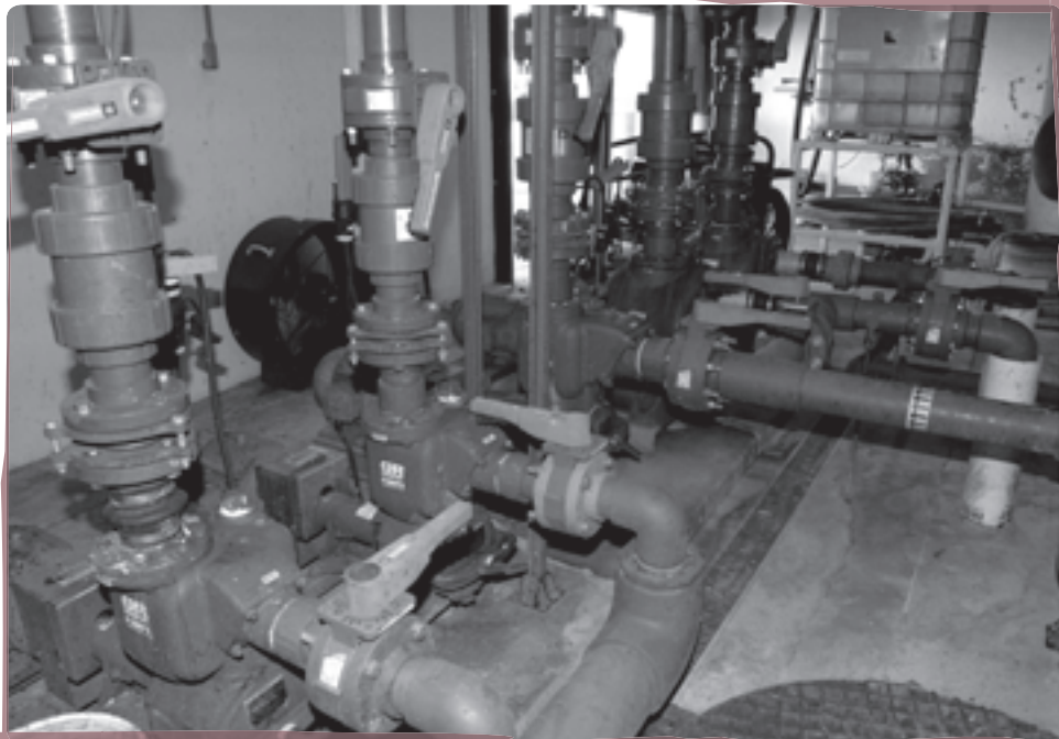
The company relied on the Super T-Series technology for several reasons, but mainly for its ability to handle solids in demanding situations.
