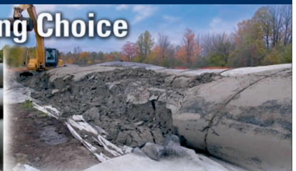
Once dewatered, the Geotube® container is opened for solids removal.
