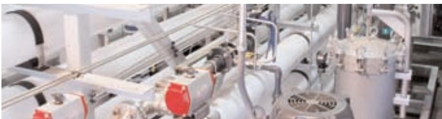
Completed RO units provide 400 gpm of treated water for the Phillipsburg ethanol plant's boiler, cooling towers and refining process.
