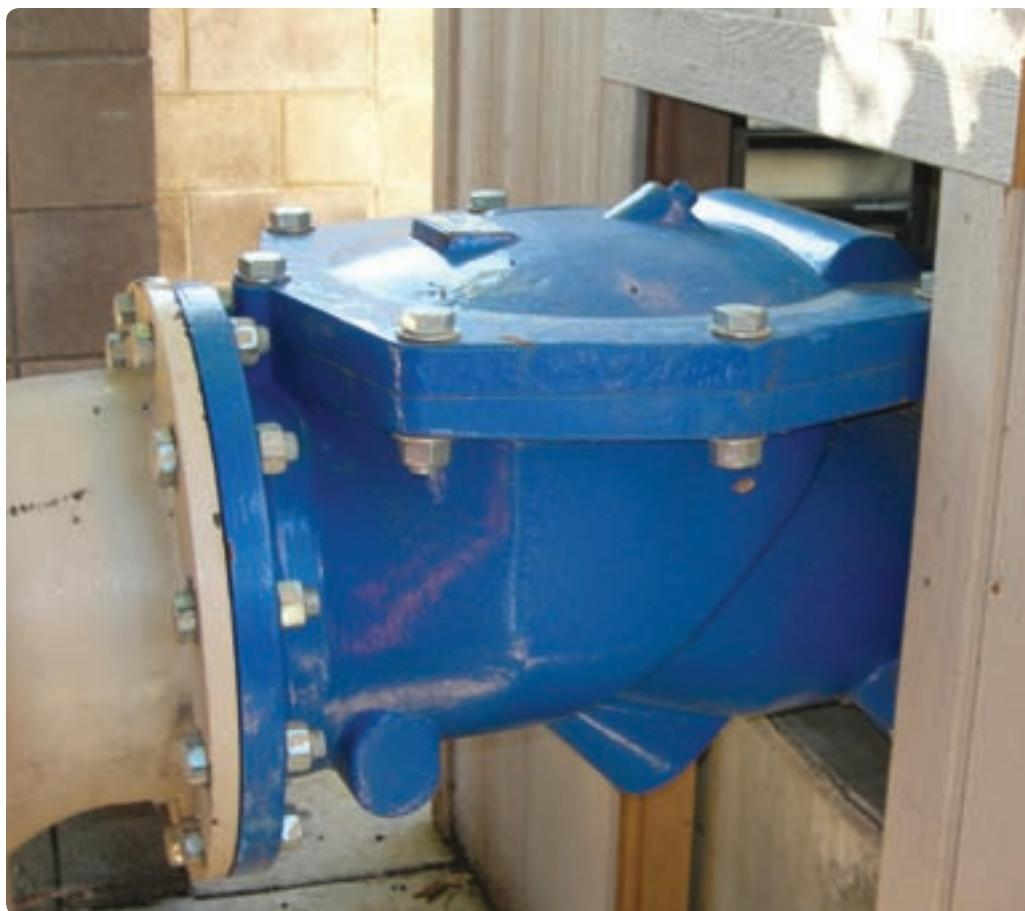
*A special kind of check valve solves the common problem of valve slam in Fresno, Calif.*
