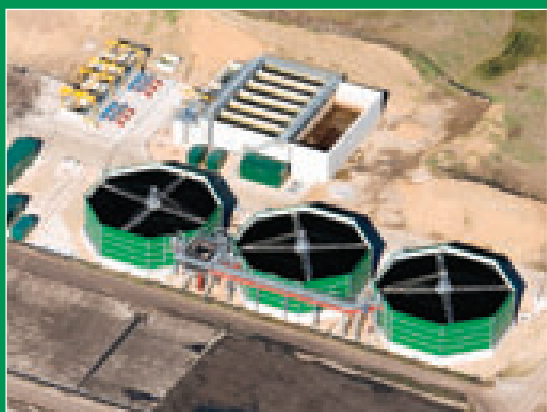
The Ashford Consent Compliance Scheme is the first of three improvement projects at Ashford WTW.
