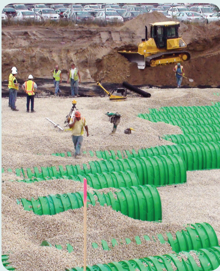
Excavation work for the 420 chambers was completed in five days.
