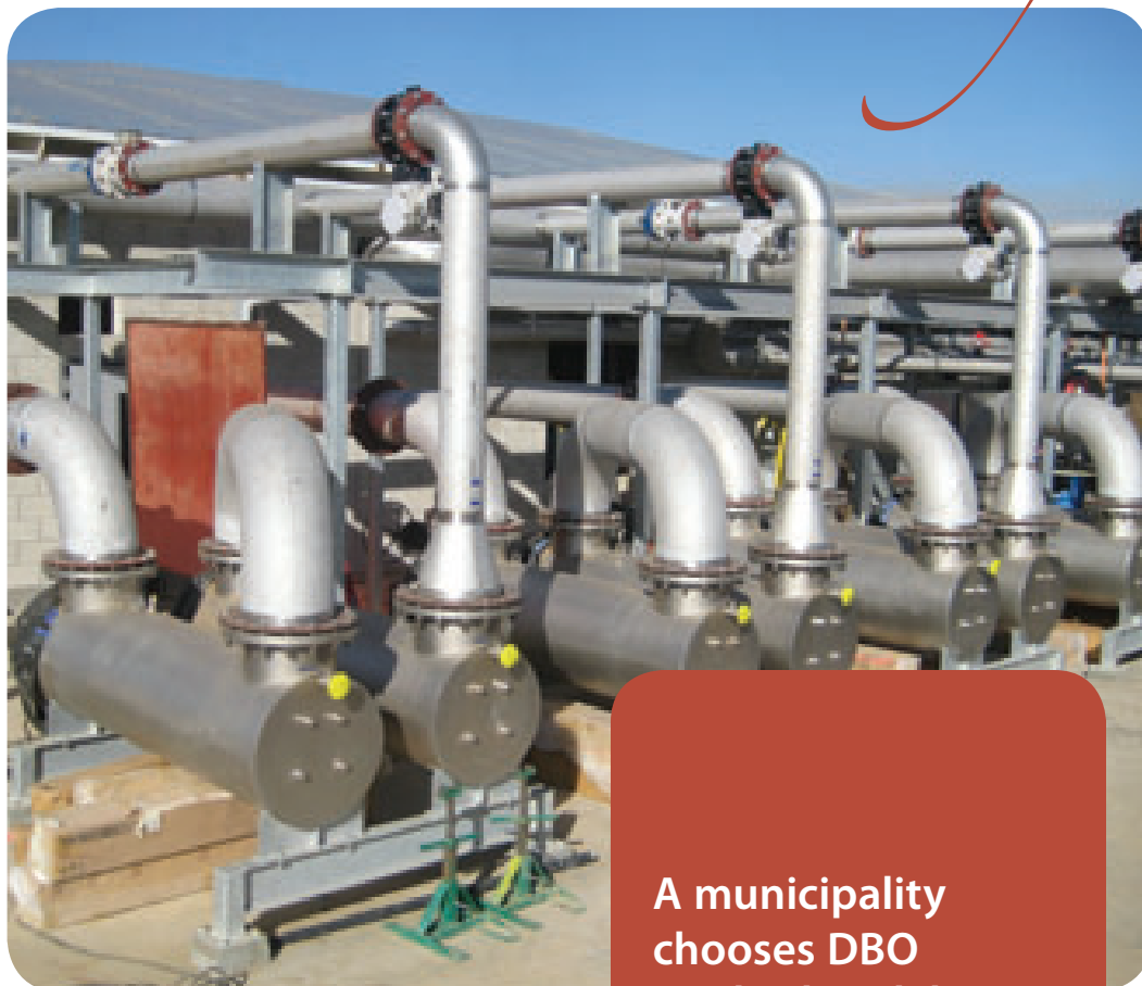
WEDCO LBX Series closed vessel UV reactors.
