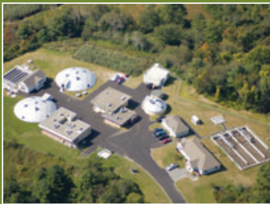
A site-specific construction plan allowed a retrofit of the facility's existing infrastructure, while maintaining treatment to meet discharge permitting standards.
