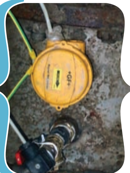
Top left: For the larger pipe, the Signet 3-2552 Magmeter adjusted to fit sizes 14 to 40 in. Bottom right: Visual site inspection of the Signet 3-2551 Magmeter.
