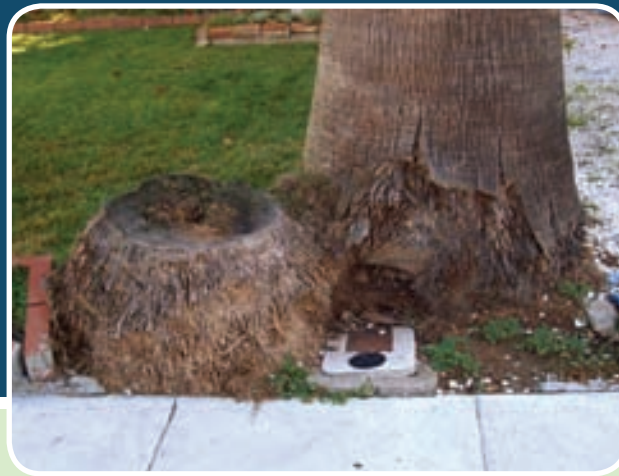
Tree roots near old meters have posed a replacement challenge, but to date, Foster City has installed about 2,000 new meters.
