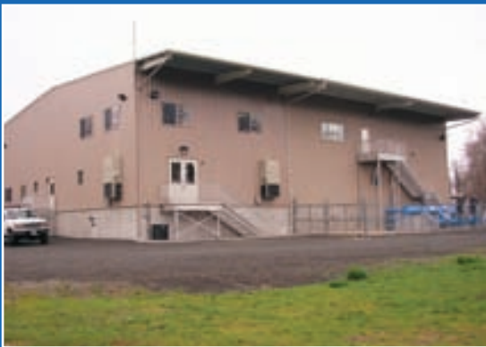
After careful consideration, the city of Cottage Grove decommissioned the Layng Creek WTP and expanded its Row River WTP.
