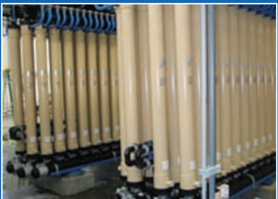
Row River WTP converted from a conventional granular media filtration process to pressurized MF membranes.
