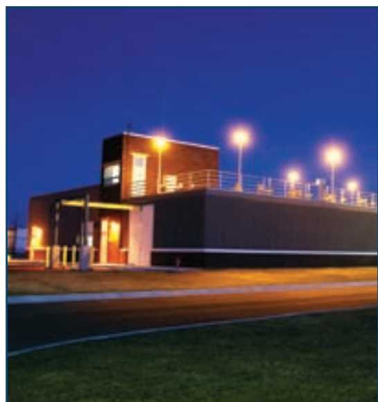
A new denitrification process removes nitrate and filters water simultaneously within the process train. The treated effluent then flows into the South Platte River.
