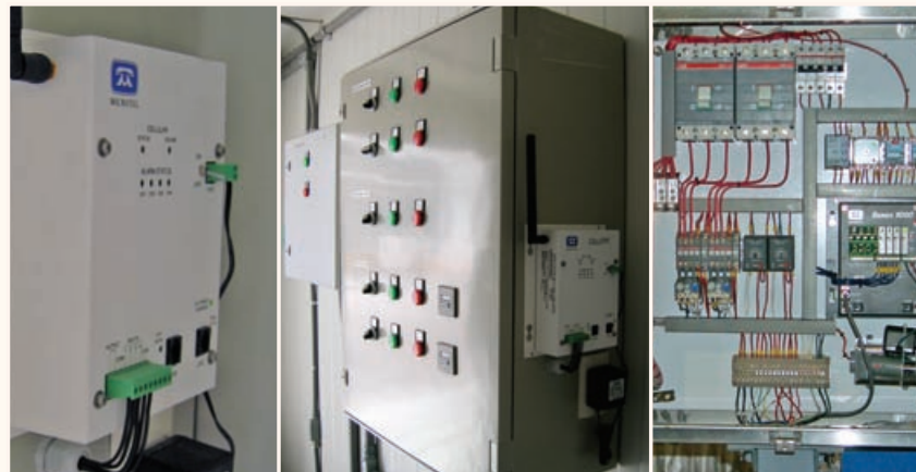
Autodialers can enhance Ethernet-based SCADA systems by providing network failure alarms.
