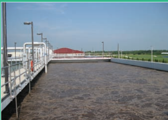
The city of St. Cloud once operated two WWTFs. Today it treats all wastewater at the recently expanded Southside WWTF.
