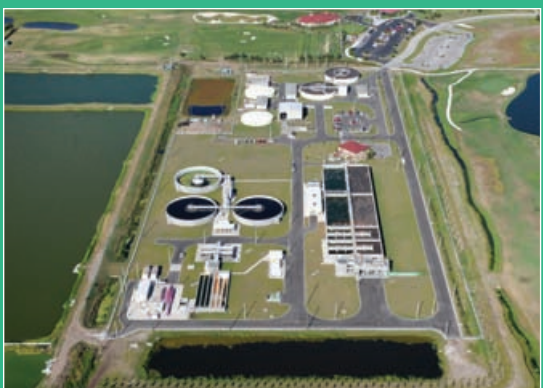
Southside WWTF is designed to accommodate additional treatment infrastructure should service demand increase.
