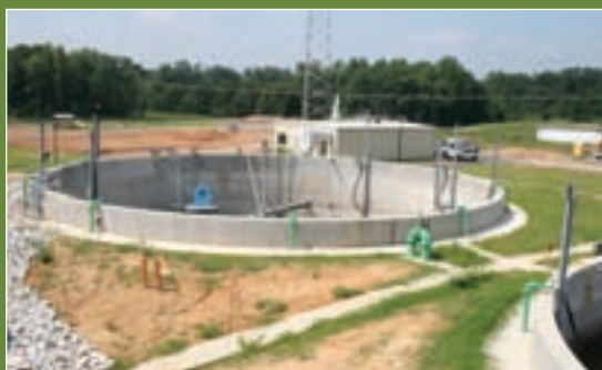
The work of new SBRs is one part of the intricate process that treats wastewater at the newly expanded HCWSA Bear Creek WWTP.
