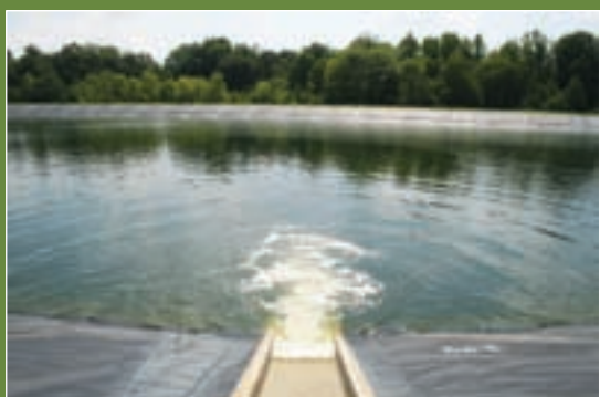
Effluent flows into the retention pond before being pumped out for spray irrigation on protected green space adjacent to the facility.
