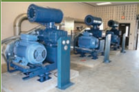
Submersible pumps send flows to the plant's headworks.
