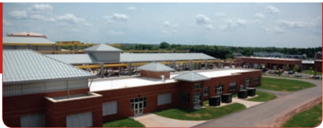
The award-winning facility includes an attractive brick panel design, extensive odor control, a visitor information center called the Aquary and park-like landscaping.
