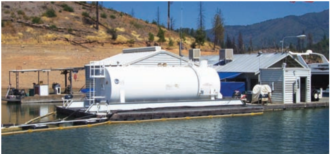
A new California regulation required that gray water no longer be discharged from houseboats on Shasta Lake; marinas are now required to provide temporary storage for it, as well as haul it off site or dispose of it in onsite drainfields.
