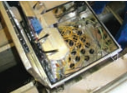
Erie WRF's new UV modules allow it to increase UV-C output without sacrificing efficiency or increasing footprint.
