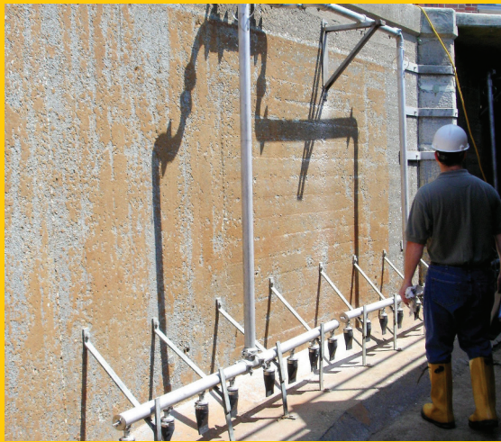
The assemblies can be lifted out, inspected and replaced without having to dewater the channel. The cradle brackets provide a guide when reconnecting the assembly.
