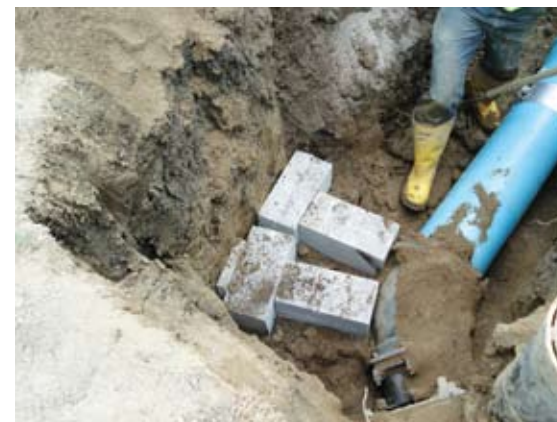
PVCO pipe has a thinner wall and is lighter than comparable materials, yet still has an HDB of 7,100 psi.
