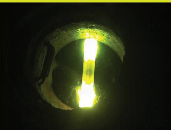
Sanitary Sewer Rehab Project No. 1 included replacing roughly 8,300 ft of sanitary sewer, 100 lateral connections and point repairs and 65 manholes.
