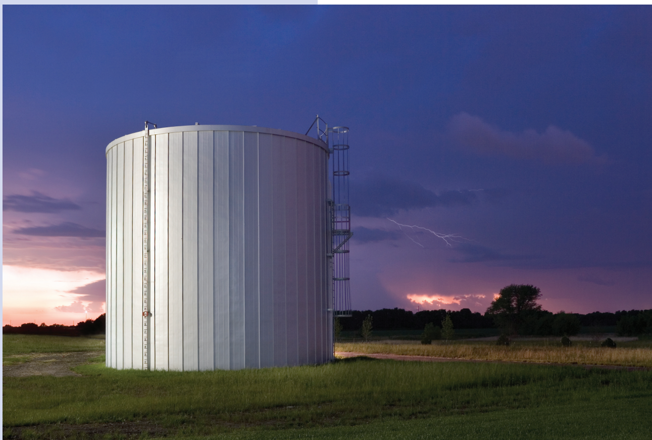
A bolted design tank uses less steel than factory-welded tanks, and thus saves 25 more tons of carbon dioxide during construction.
