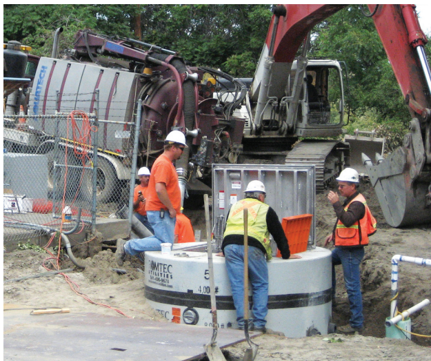
Installation of the new pump station took place in July 2009.
