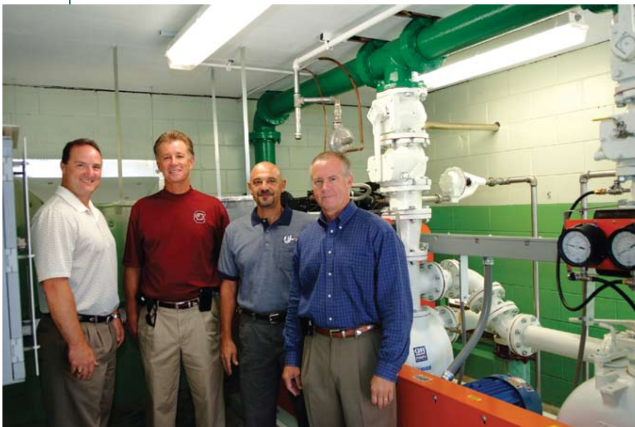
From left to right: Todd Ritchie, municipal sales engineer for TenCarva Machinery Co.; Frank Emminger, general manager for DuPriest Construction; Joe DeVito, BJWSA director of field operations; and Robert Horner, principal for HEG Eng. Consultants.
