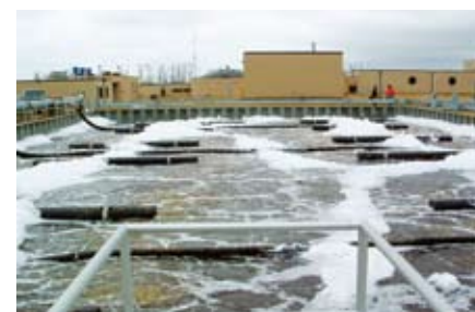
The ActiveCell MBBR process was selected after a five-month pilot program; it has the ability to operate on a single pass without the need for postclarification. The system provides high-rate nitrification and requires minimal operator attention.
