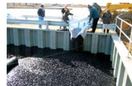
The ActiveCell MBBR process was selected after a five-month pilot program; it has the ability to operate on a single pass without the need for postclarification. The system provides high-rate nitrification and requires minimal operator attention.
