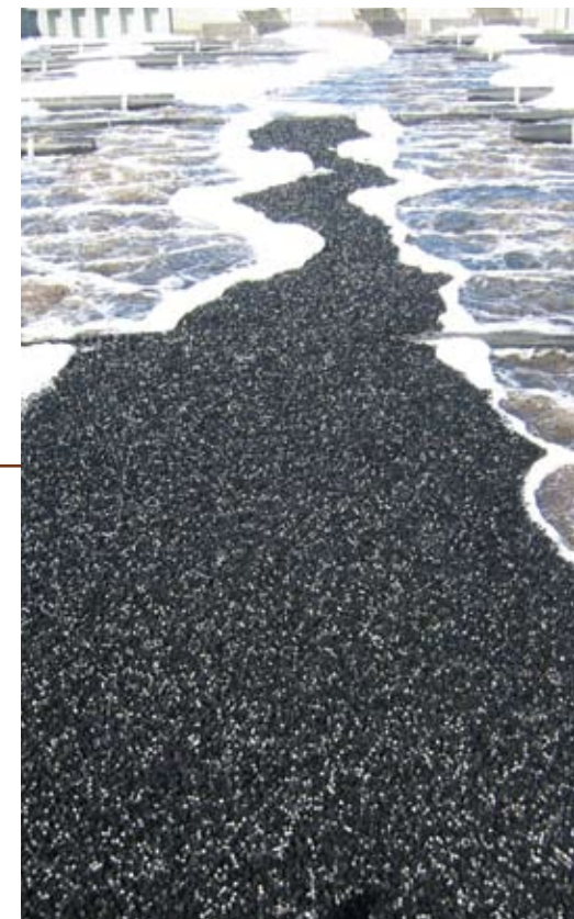
The ActiveCell MBBR process was selected after a five-month pilot program; it has the ability to operate on a single pass without the need for postclarification. The system provides high-rate nitrification and requires minimal operator attention.
