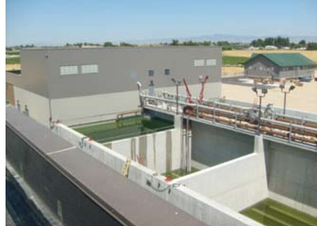
One of two biological treatment trains and the membrane system process building.
