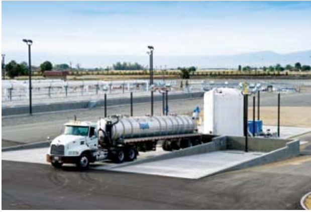
Truck unloading at grease-receiving station. Grease is added to digesters to increase gas production.
