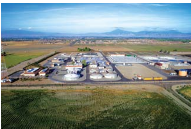
The upgraded Bakersfield Wastewater Treatment Plant 3.
