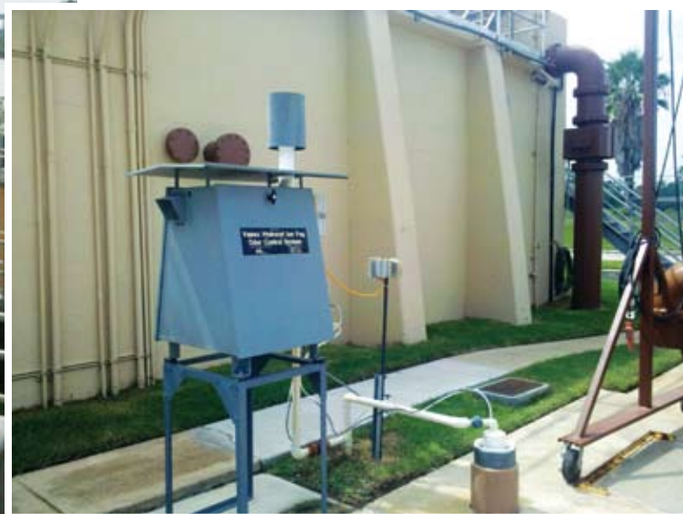
Unlike a scrubber system, O-MEGA systems eliminate the need to withdraw odorous air from the structure and pass it through a separate odor control scrubbing process.
