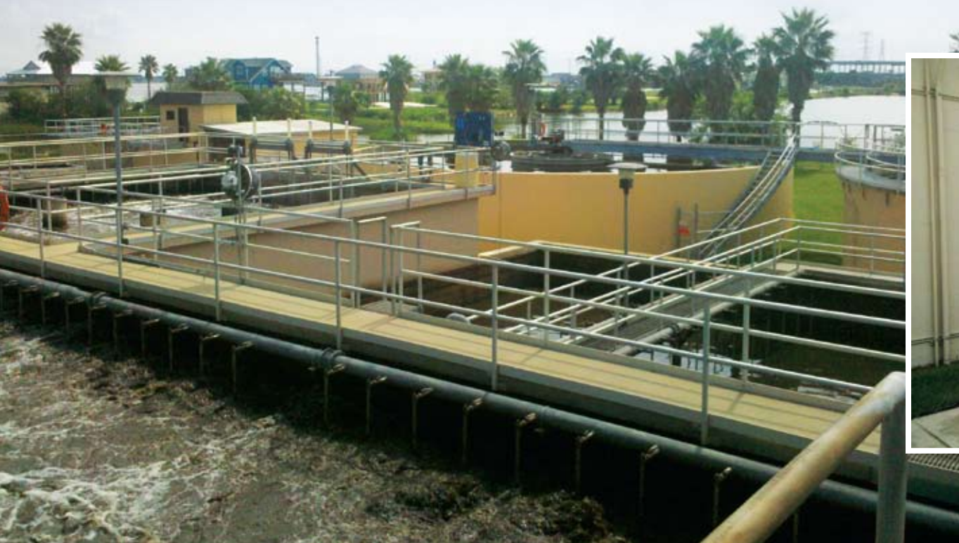
Unlike a scrubber system, O-MEGA systems eliminate the need to withdraw odorous air from the structure and pass it through a separate odor control scrubbing process.
