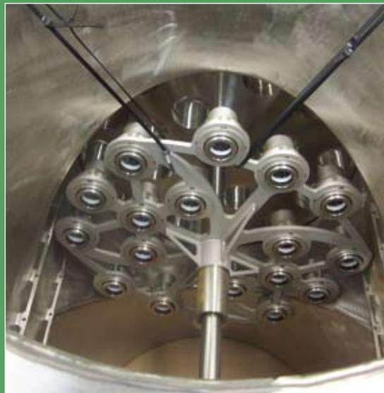
Each of the 30-in.-diameter UV light units at the Neshaminy plant can remove up to 90% of algae in water.
