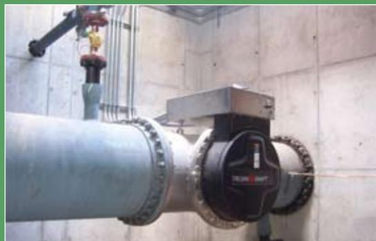
The UV lamps are kept at peak performance by the ActiClean system, shown here, which slides over the quartz sleeves containing the lamps.
