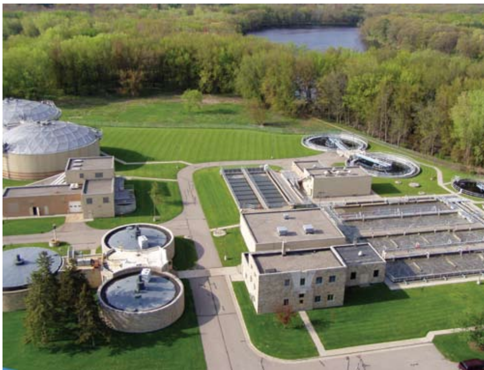
The Stevens Point WWTP treats an average of 3 million gal of sewage a day.
