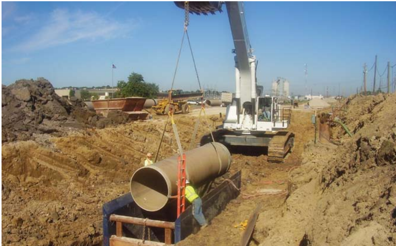
CCFRPM pipe and RCP were specified for this project.
