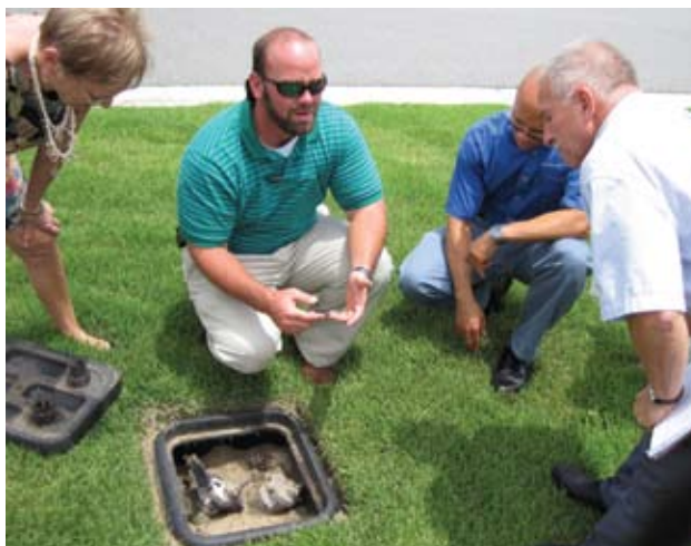
District staff members inspect the irrigation system at a potential Florida Water Star home.
