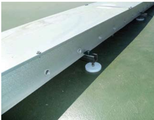
The magnetic solution proved a viable alternative to welding and allowed for a much less invasive procedure.
