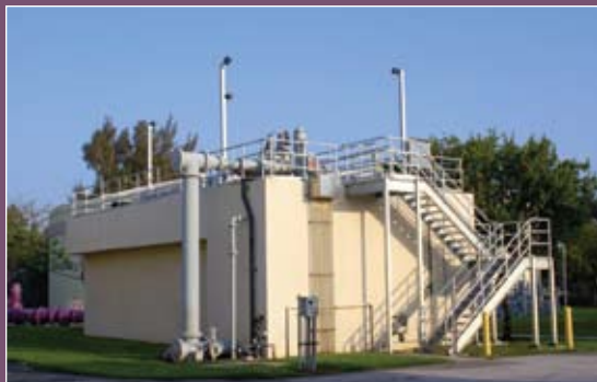
Upflow sand filters are key components of the facility.
