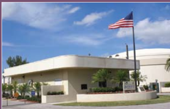
The OASIS reuse program protects the city’s potable water wells.
