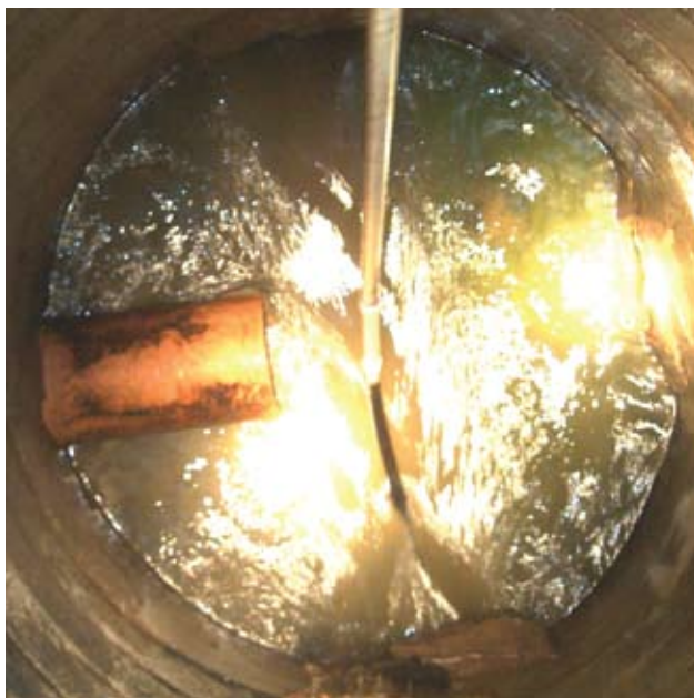
Installation in a manhole.
