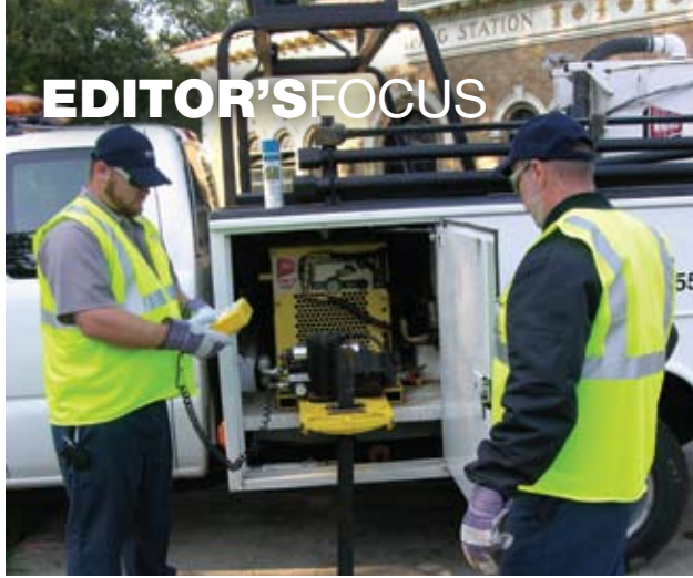
Wachs Water Services staff performing a valve assessment for the city of Baltimore.
