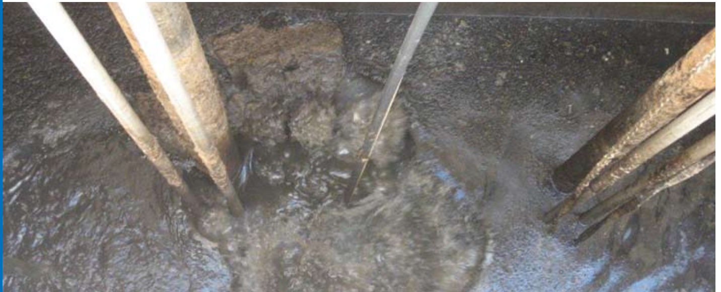
The plant's new mixing technology works by allowing a burst of compressed air at the base of the well to break up the cap.
